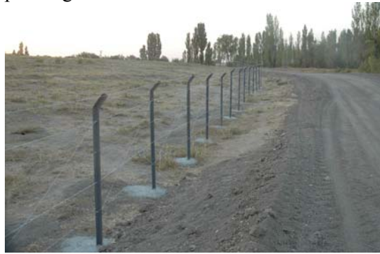
With funding from the Global Heritage Fund, a fence was constructed around the West Mound.
