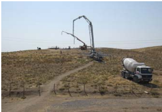
Figure 12: Staged concrete pourers
