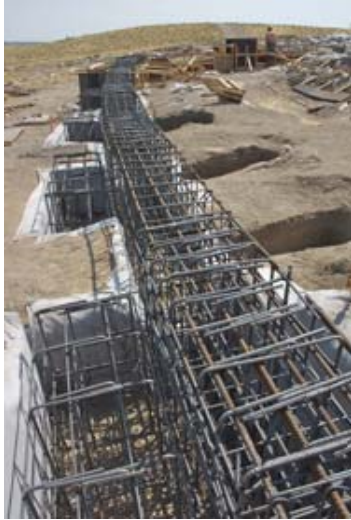
Figure 11: Lined and reinforced foundations for the Shelter.
