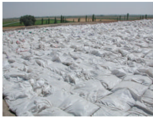
Figure 66: 4040 Area backfilled with sandbags
