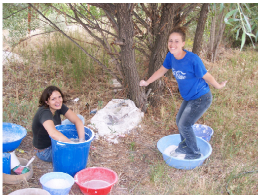
Figure 134. Wall plaster preparation.
