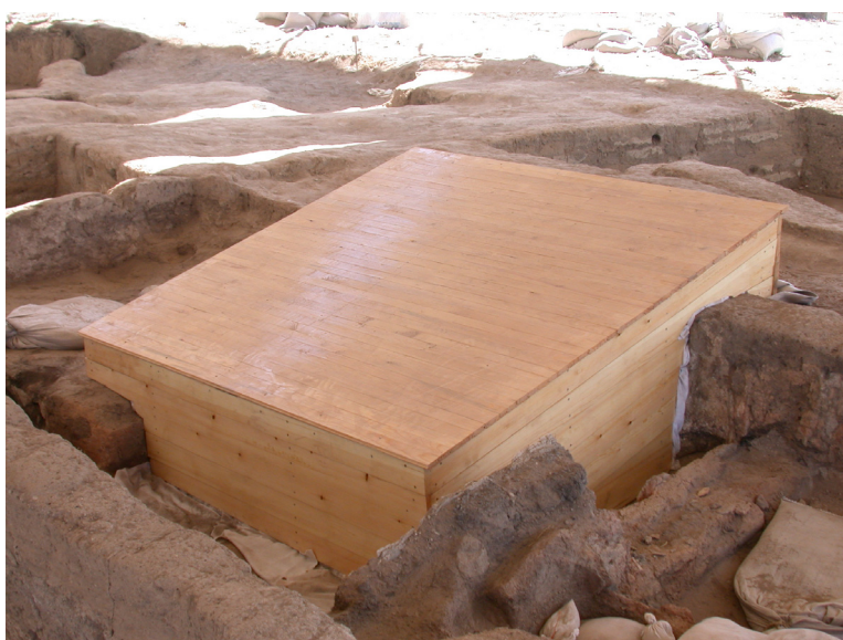
Figure 118. The wooden box after construction
