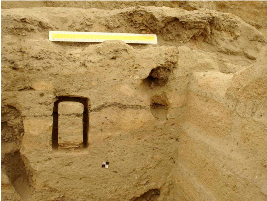
Figure 168: Non-plastered exterior wall face and surfaces of Building 53, South Area. Looking S, scale = 30 cm. Sample 11379.04.
