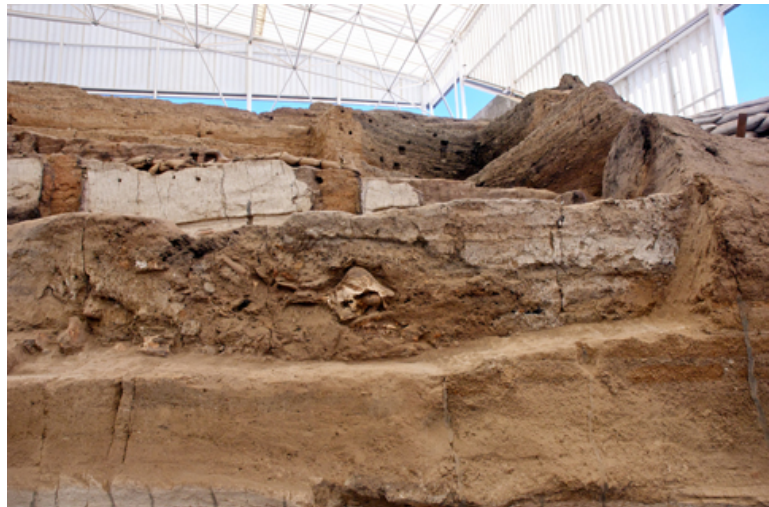
Figure 3.9. East facing through B.80/B.76 walls, clearly showing 'between wall fill' (19802).
