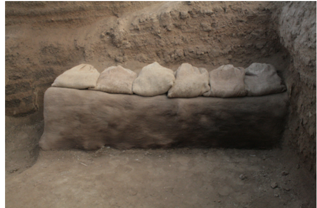
Figure 17.1. Features 223, 350, and 246 after application of new capping
